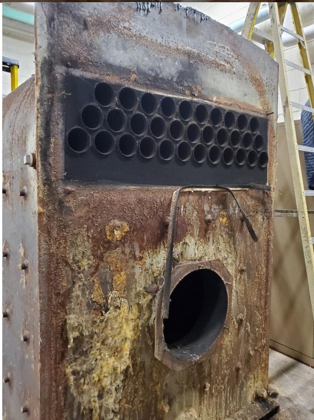
**Removal of old fuel oil boiler in preparation for new propane boiler.**
