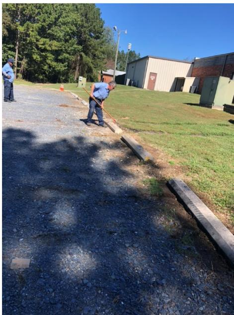
The front wall of Building 500 has some water issues. Upon investigation, it was found that the front foundation seal is failing. To repair this, the maintenance crew will dig along the brick portion of the wall (grassed area), install drainage pipe along edge, and back-fill with gravel. The stucco walls along the front sidewalk also requires repairs.
