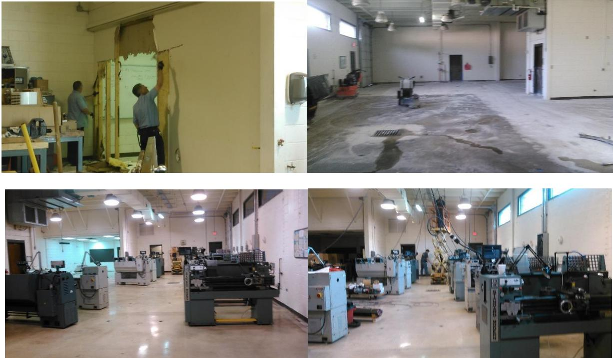
The wall between Rooms 507 & 508 has been removed to accommodate the lecture and physical training for Department of Correction employees. After the wall was removed, carpet was removed, the concrete floor ground, dyed, and polished.
